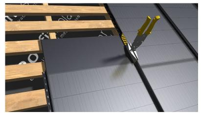
Step 9. In corners, where 4 modules meet, use pliers to tighten the upper right side lock before next module is installed.
