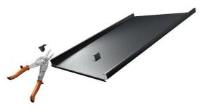
**Step 1.** Prepare the top metal part by cutting the seams and forming a backbend.
