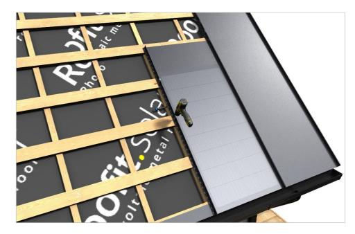
After locking the seam, **Roofit**.solar module is screwed into the place using flat-head screws.
